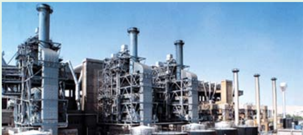
An overview of a thermal power plant
