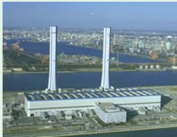
An overview of a thermal power plant near Tokyo, Japan
